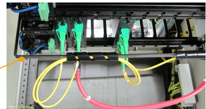
CH3000U-FM-01 Fiber Routing Shelf under the CH3000 Chassis
